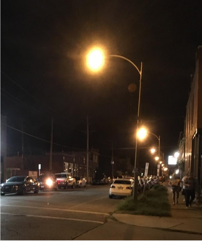
Figure 88: Current lighting in the Macklind Business District
