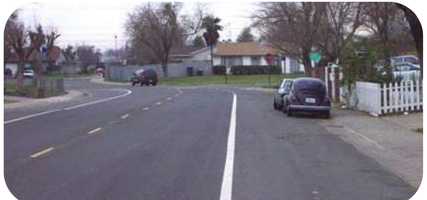
Figure 70: Example of edge line striping, which visually reduces roadway width
