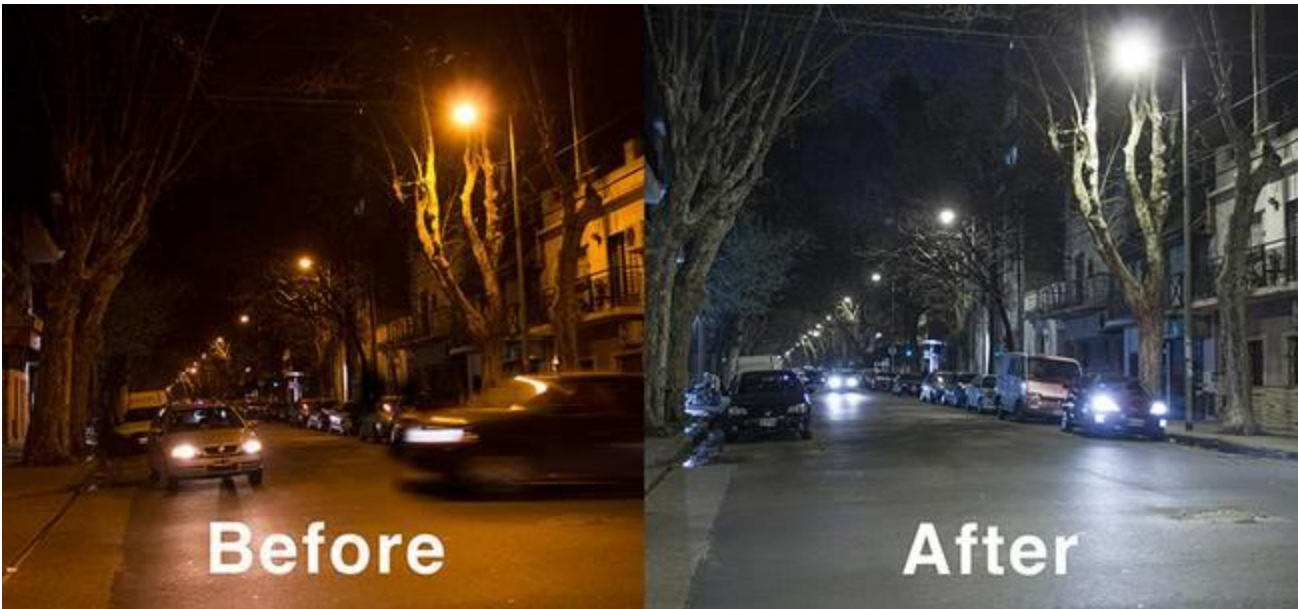
Figure 89: Before and After LED lighting installation
