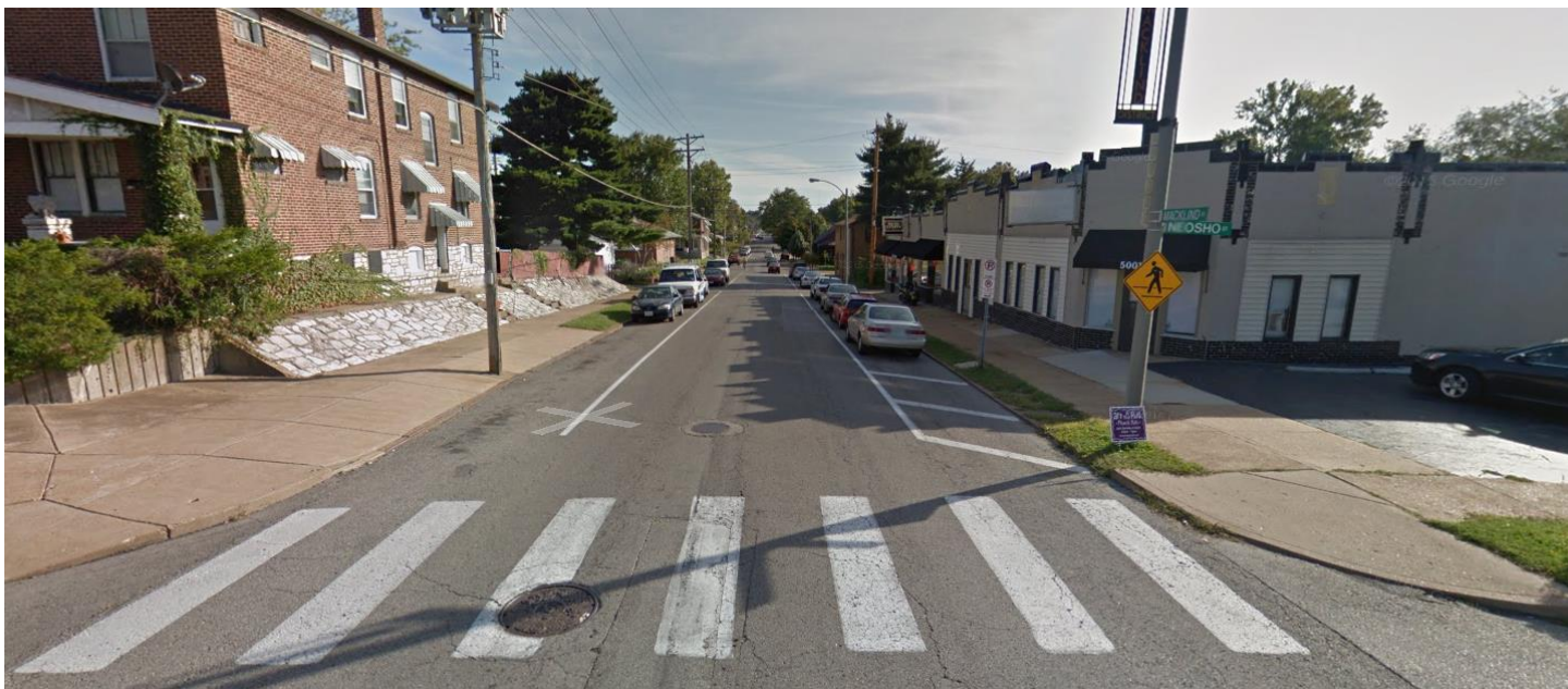
Figure 45: Continental crosswalk across Macklind Ave. at Neosho St.
