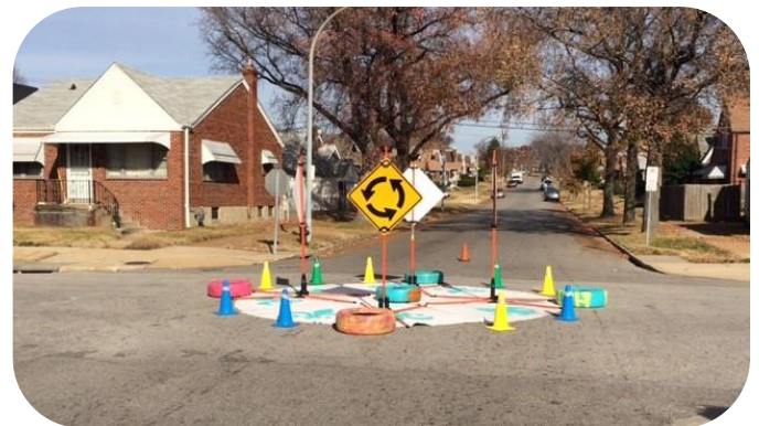
Figure 79: Example of a pop-up traffic calming circle
